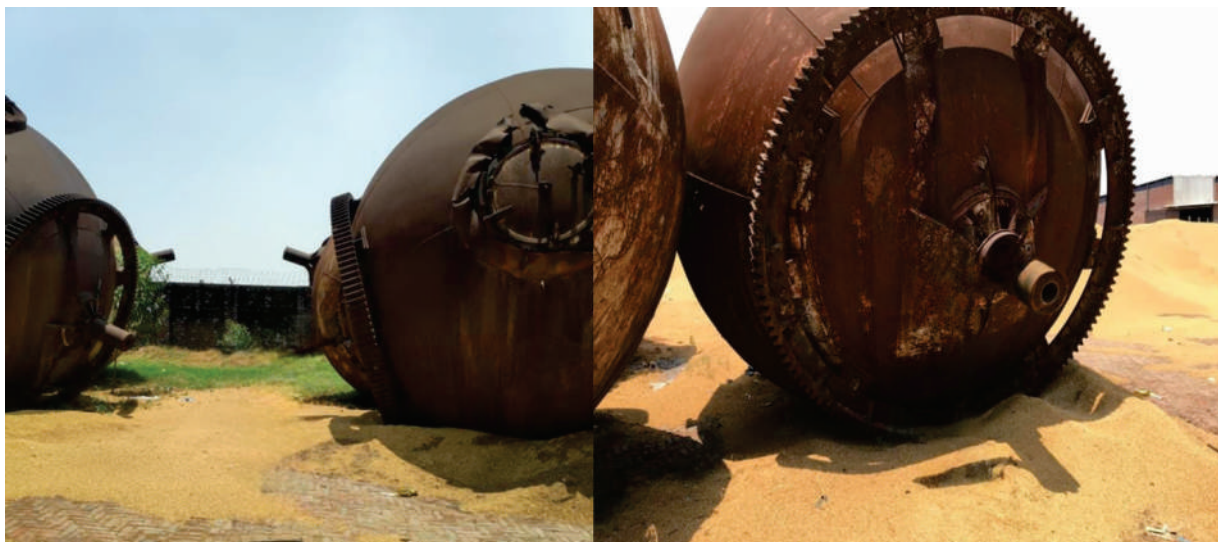
Fig. 2: Dismantling of digestors at pulp and paper industries not having CRP.
